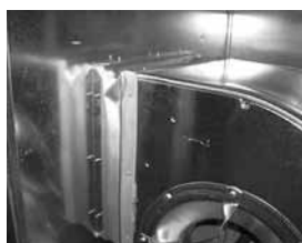
◀ Flexible connection between cabinet panel and fan outlet
