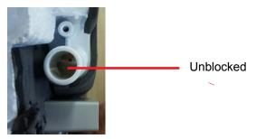
But for AWSI-HBV16/18/24 and WSI-HBV30 indoor untis the middle of the left drain is blocked, so first need to knock off the middle of the blocking piece and take it out to avoid noise when the unit is running. Then install the drain pipe.
